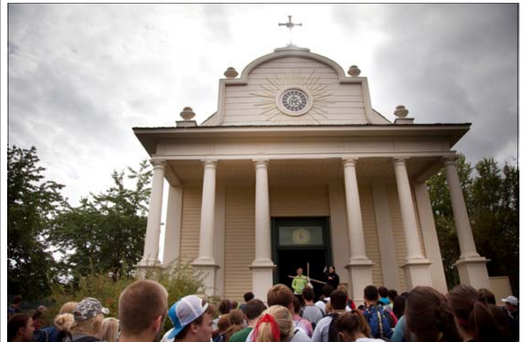
On Sept. 17, the 43rd annual Pilgrimage retreat will conclude at the Sacred Heart Mission, the oldest standing building in Idaho. The campus community is encouraged to attend.
