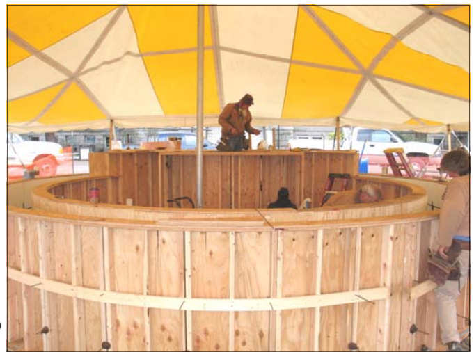
Wooden forms are readied for the reflecting pool walls.
