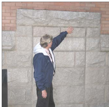
Mac McCandless traces the outline of a former door on the east wall of the southwest corner of the Ad Building.
